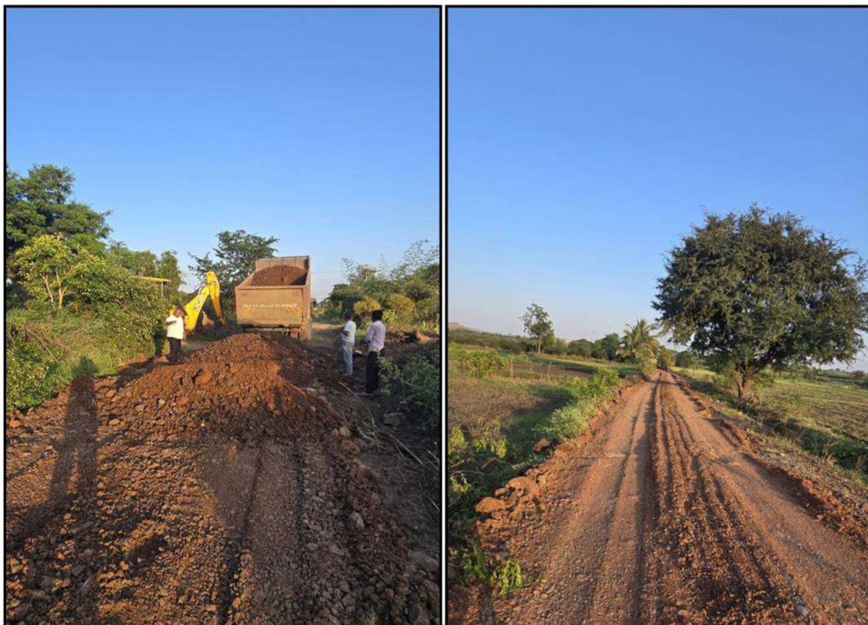
Construction of Panand road at Village Sonori
