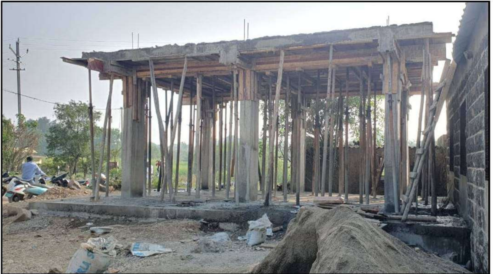
Construction of toilet unit at Z P School Village Tekwadi
