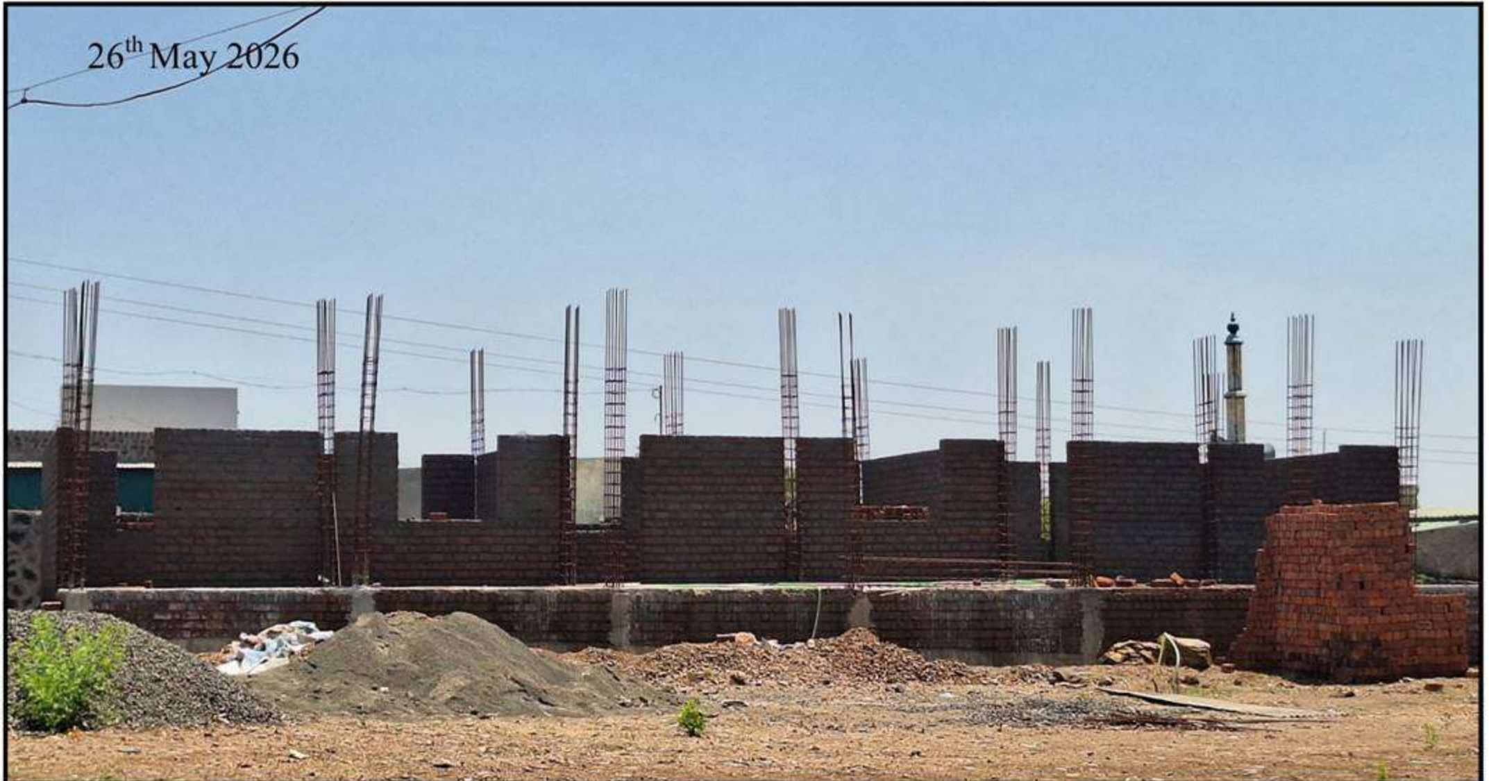
Construction of School building at Village Khatgun
