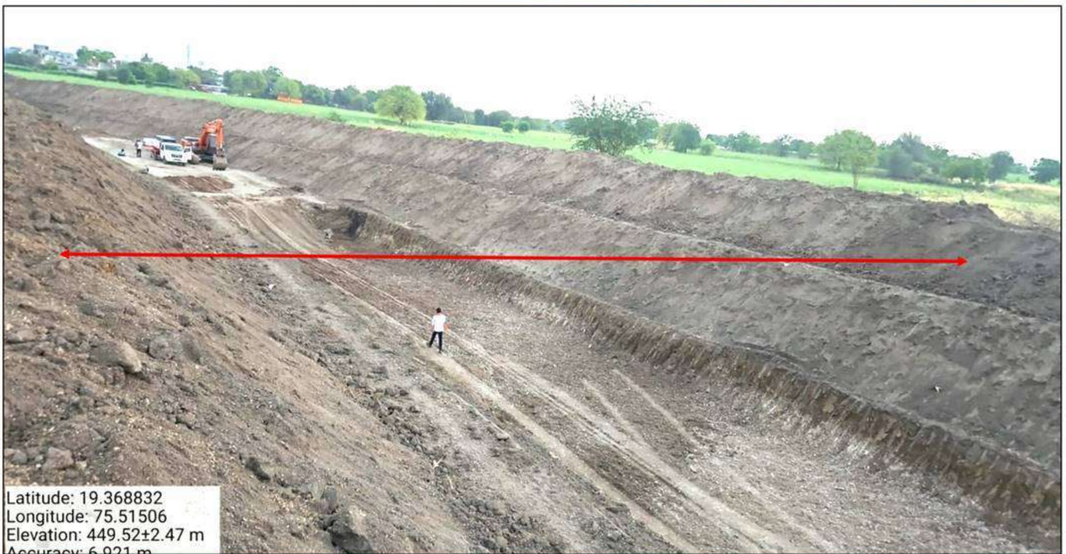
Desilting of Kambri river in Kambi village
