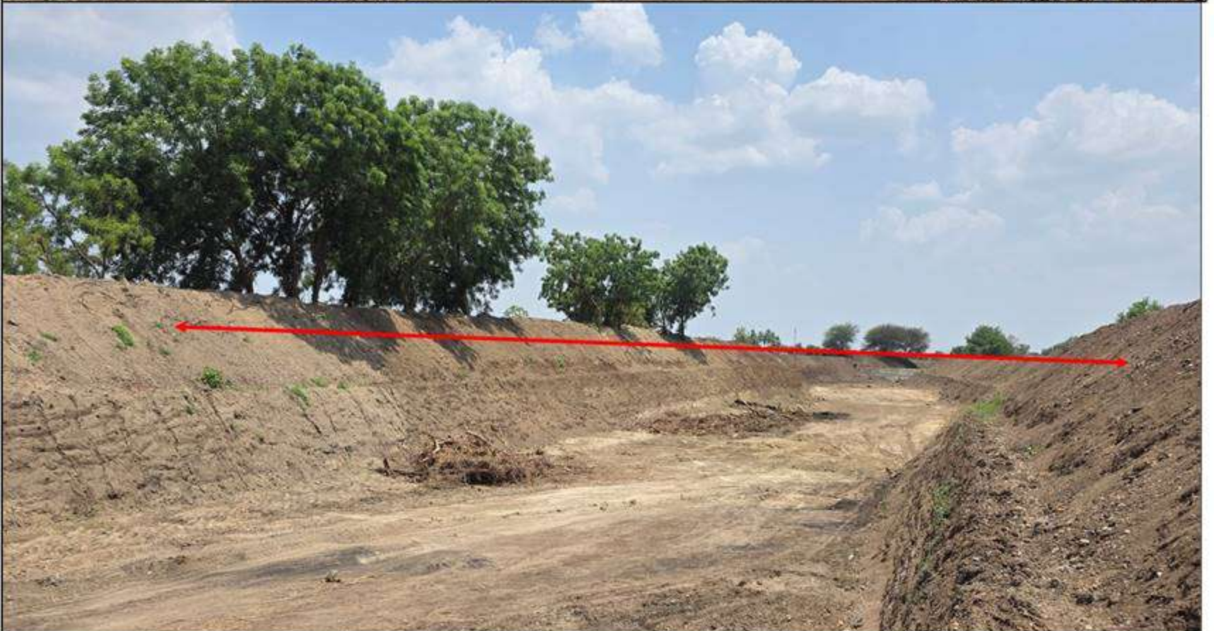
Desilting of Lendi bandhara in Gaikwad Jalgaon village
