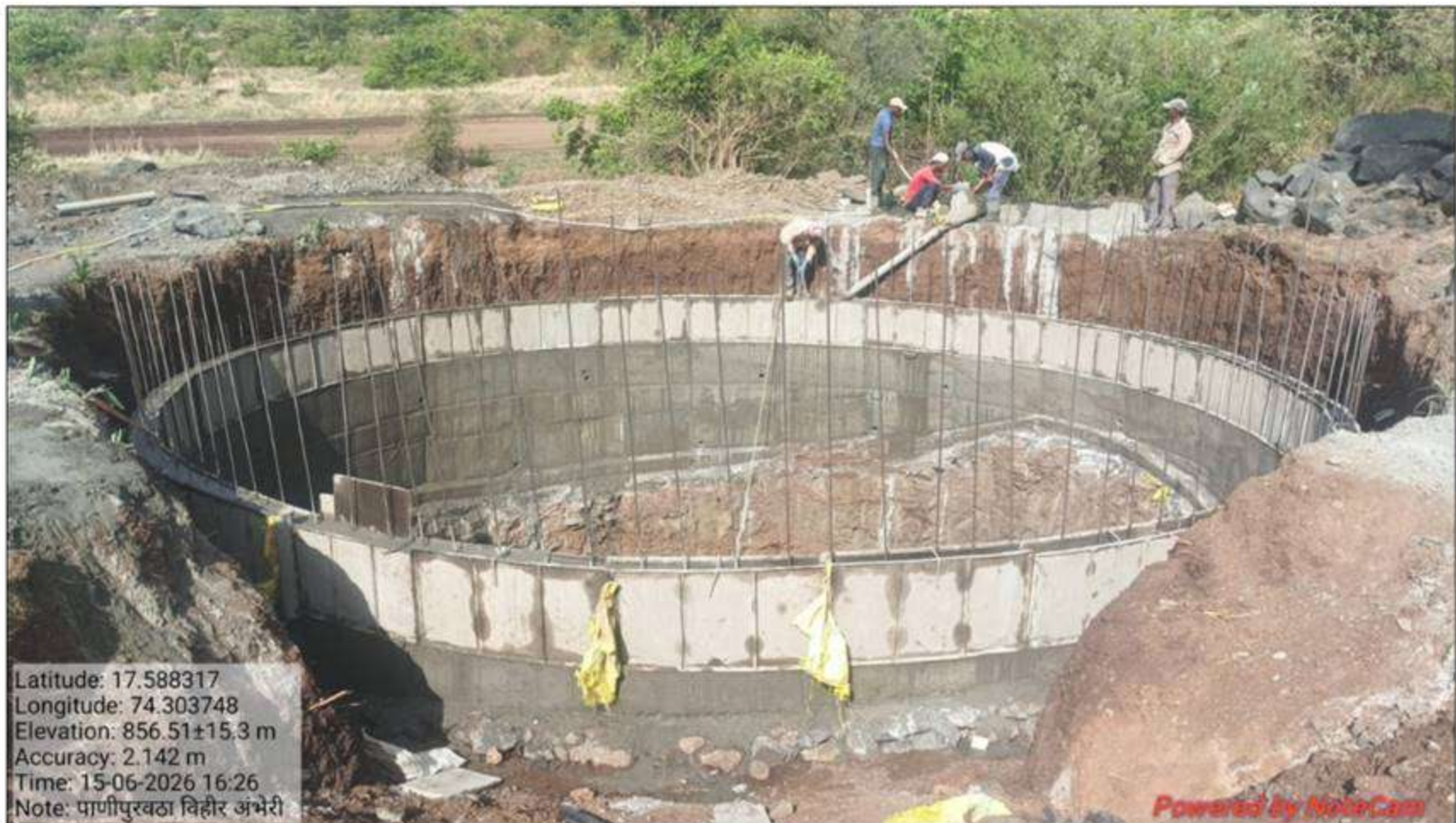
Construction of Open well for drinking water at Ambheri
