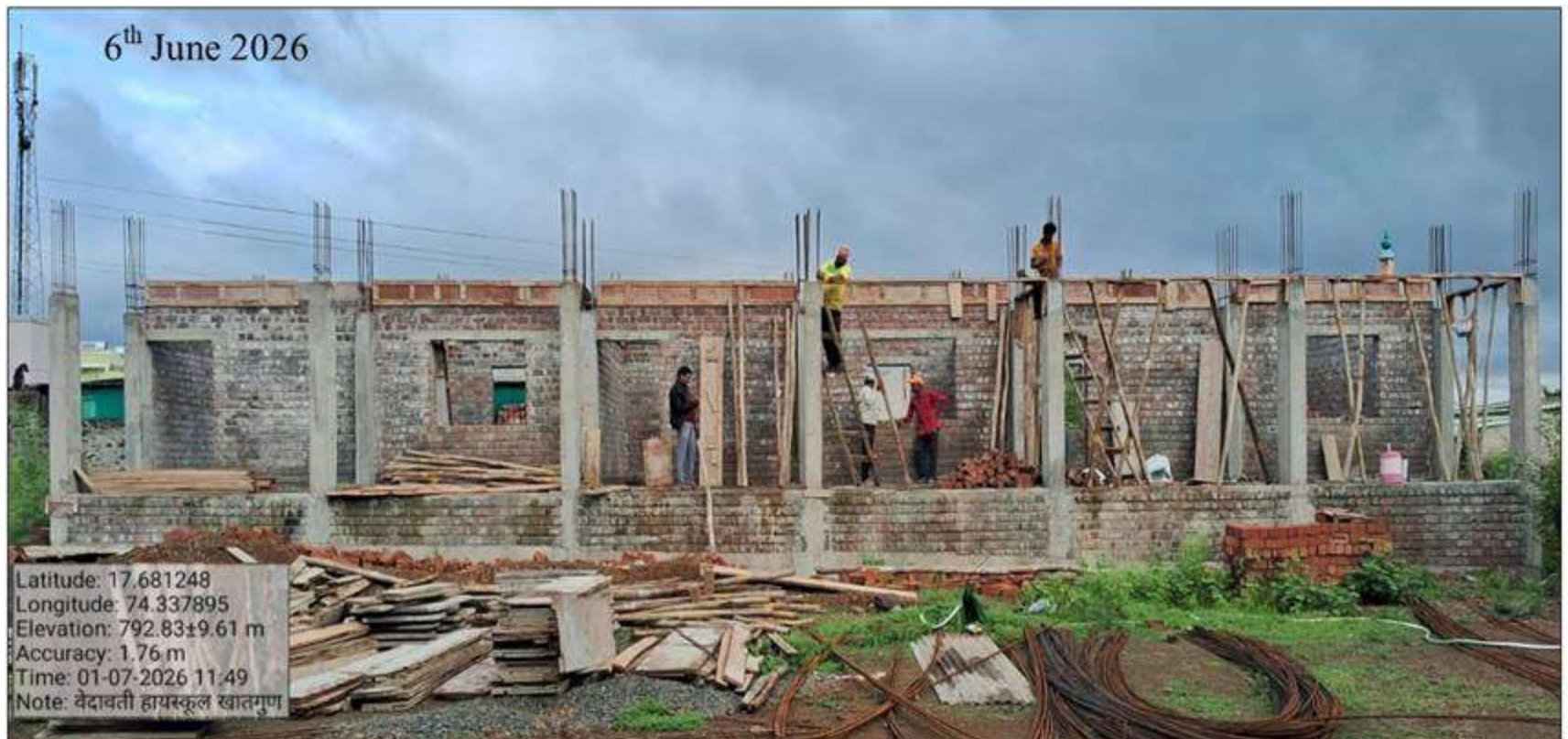
Construction of School building at Village Khatgun
