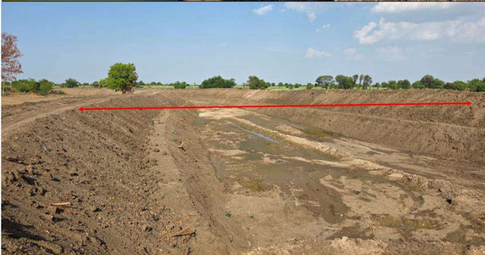
Desilting of Kambri river in Kambi village
