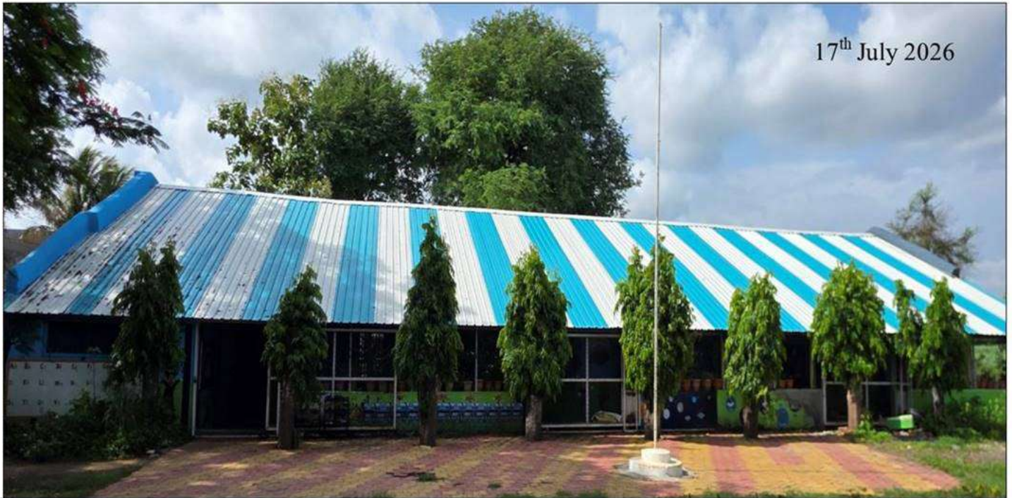
Construction of Steel sheet roof work at Z P School Village Patkhal
