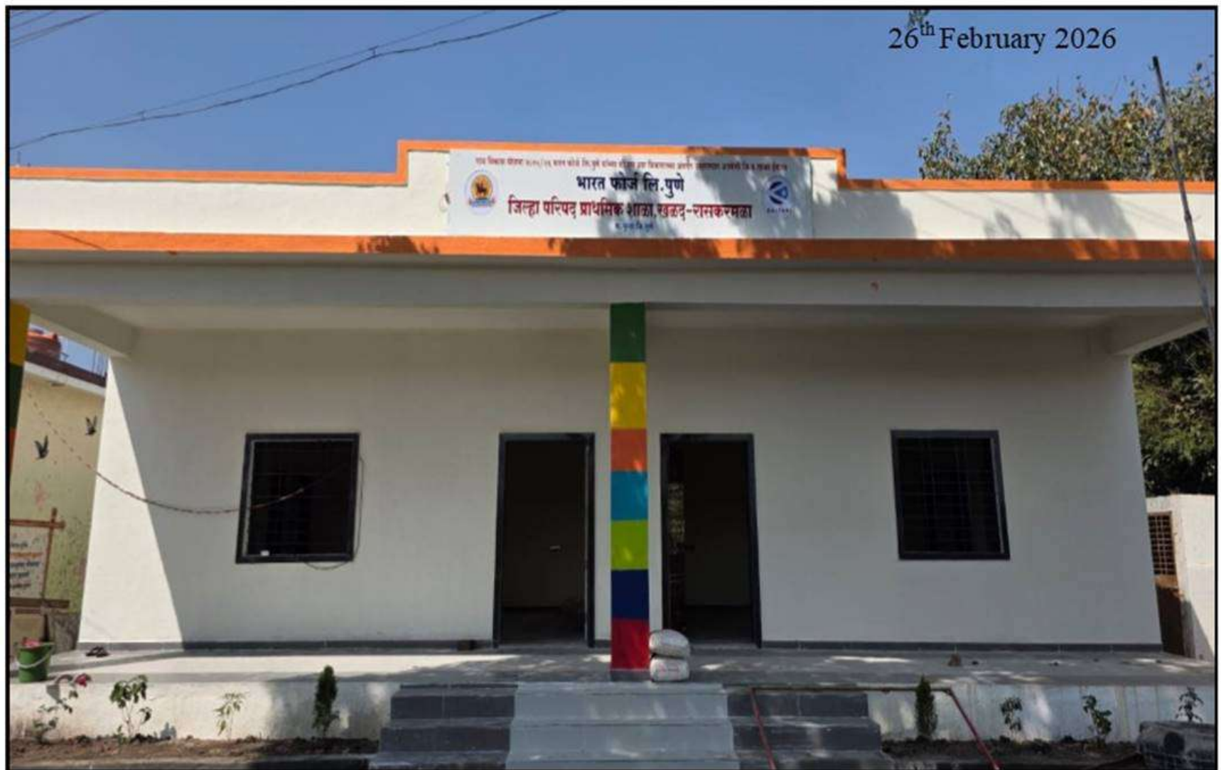
Construction of School building at Z P School Village Khalad
