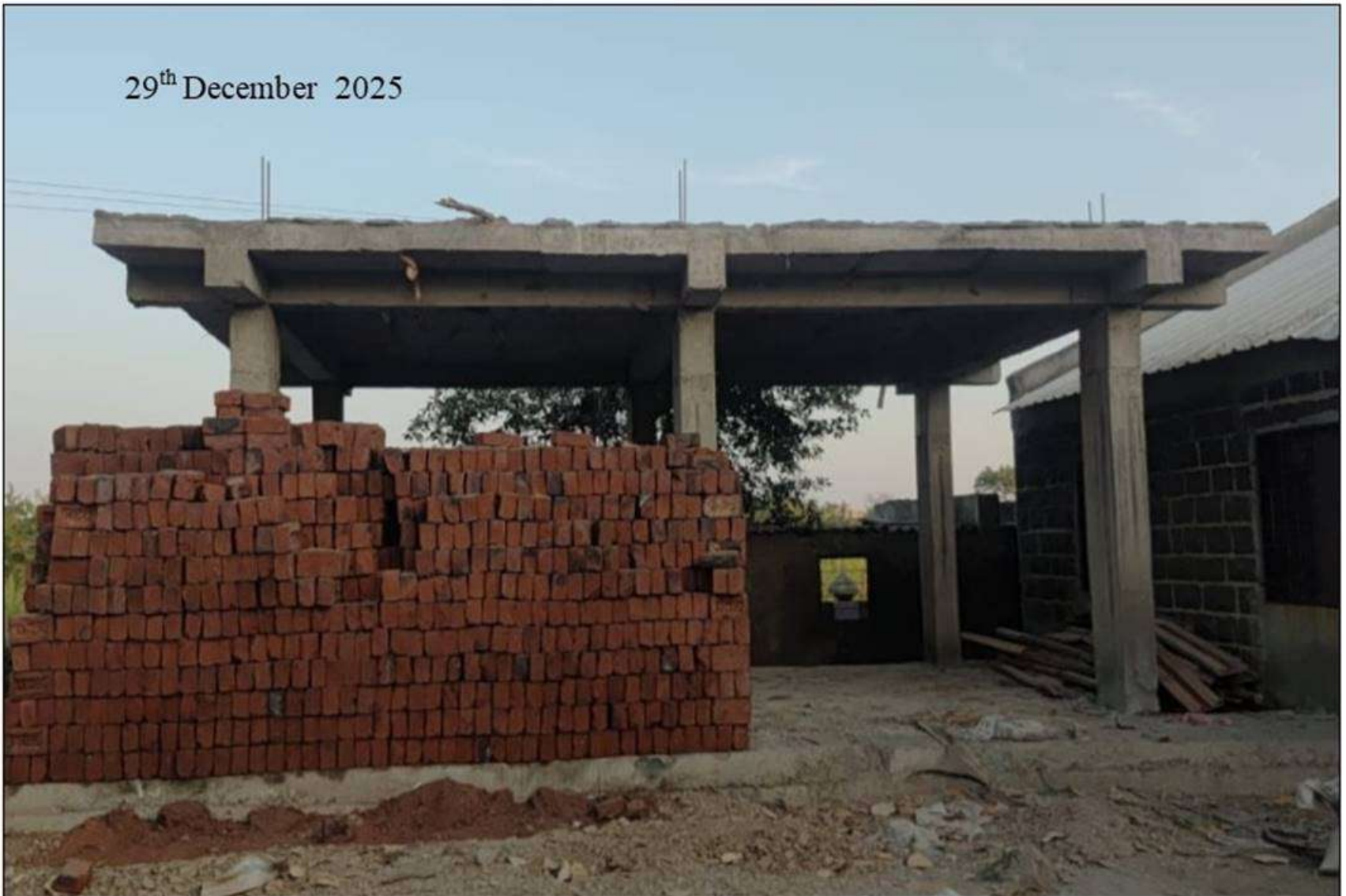
Construction of toilet unit at Z P School Village Tekwadi
