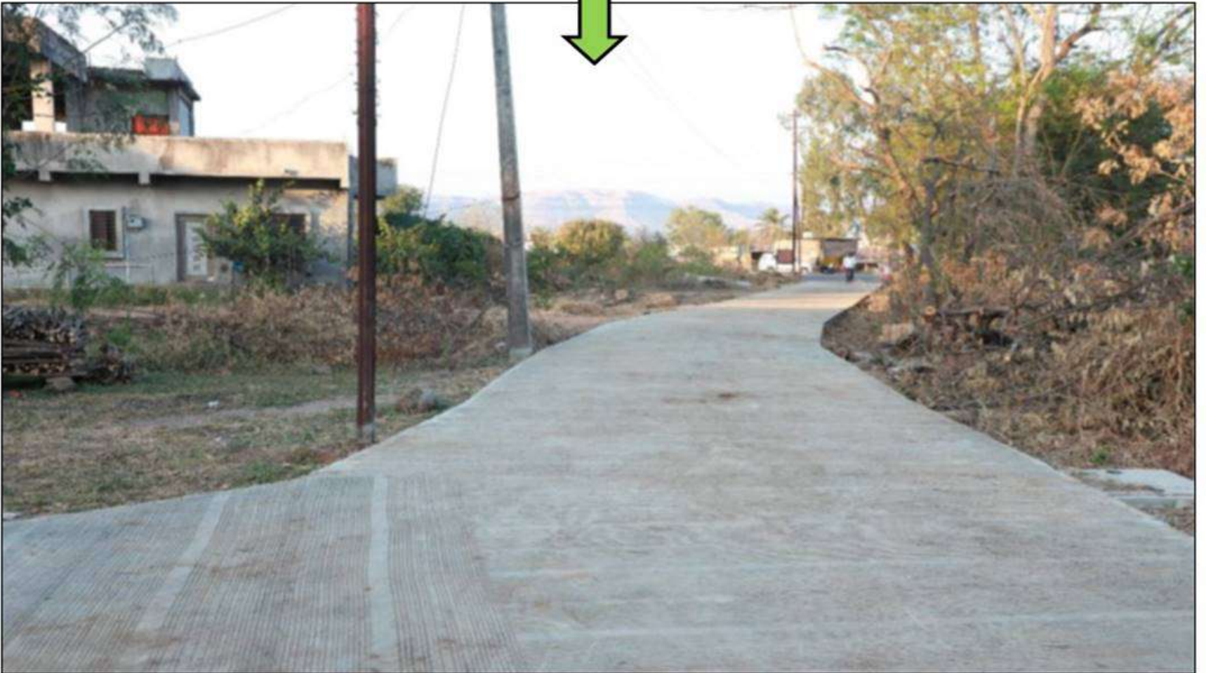
Construction of internal concrete road at Village Kole.
