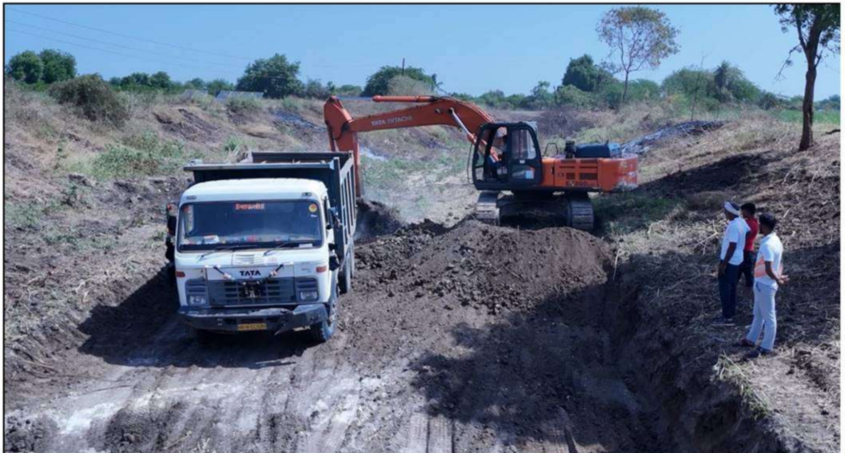
Desilting of Rajpure-Deshmukh bandhara in Balamtakali village
