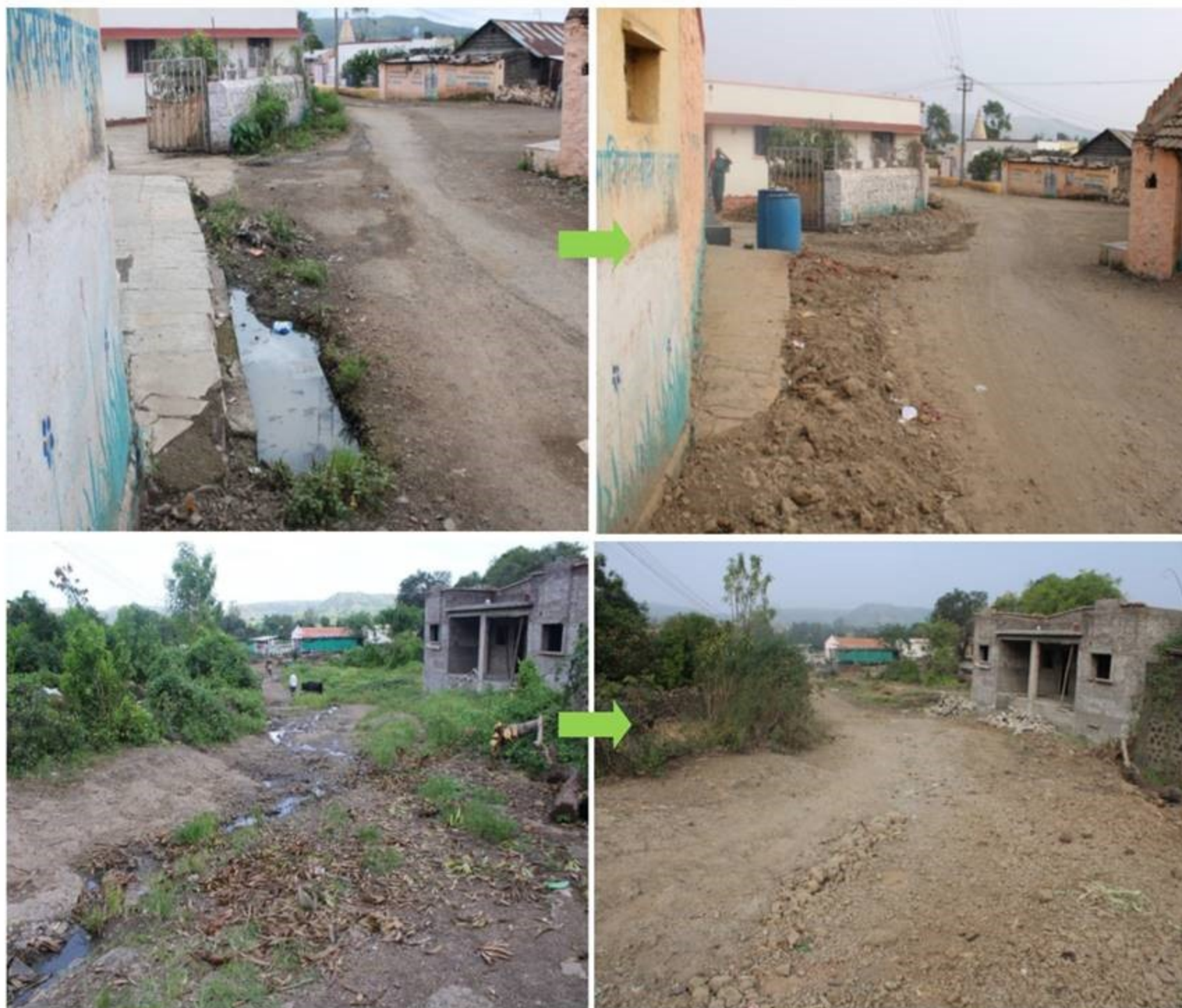
Construction of internal gutters works at Chilewadi
