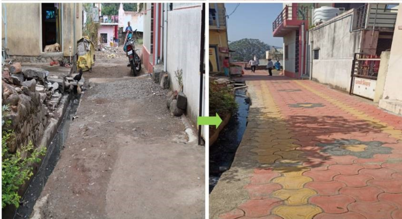
Construction of internal pavers roads at Nagzari
