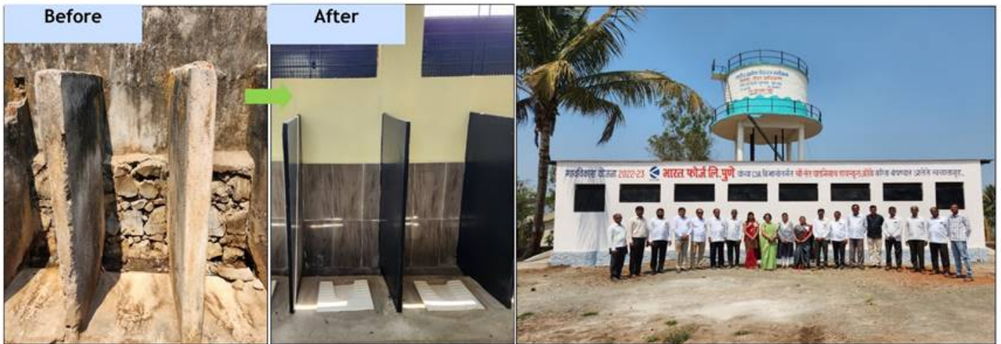
Construction of toilet unit at Gadagenath school, Village Kole
